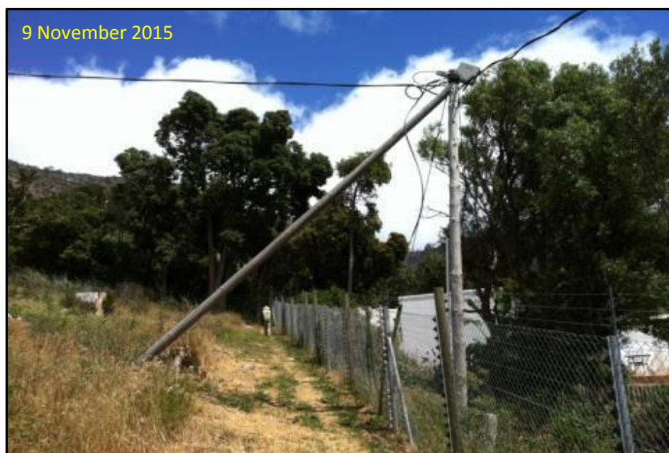
Figure 15: Telephone poles over the Zwaanswyk Fence act as a ladder for baboons to hop over the fence.
